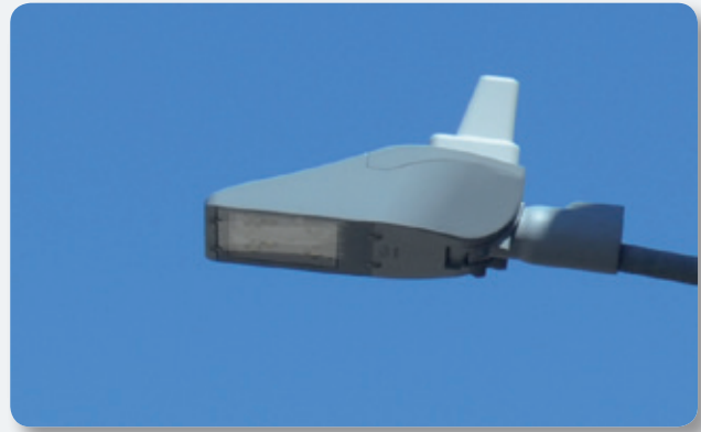
Nodo STELARIA instalado en luminaria LED | STELARIA node installed on a LED luminaire
